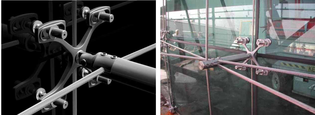
Fig. 6 Computer Rendering of the Final Spider Design and Finished Components in the San Jose Mock-Up
